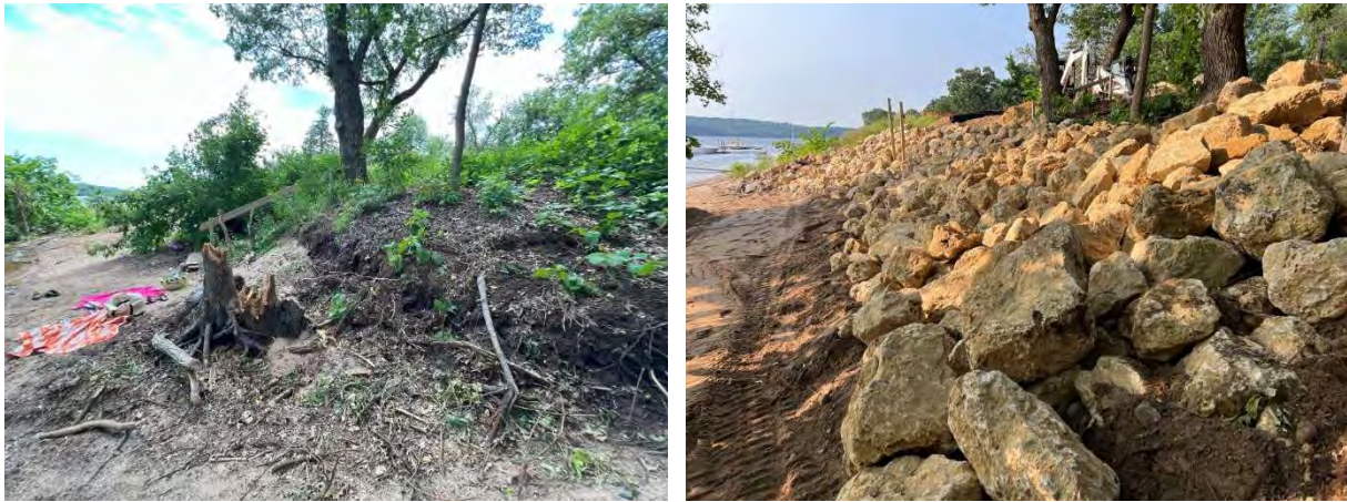
[Above] South Beach stabilization before (left) and after (right)
